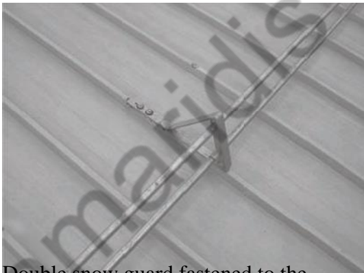
Double snow guard fastened to the purlin by means of two screws.
