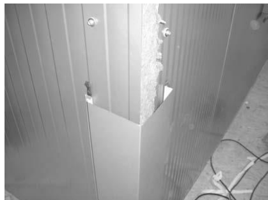
The industrial and thus more economical option with visible fixing lugs. Again, Type 4 sealing tapes must be installed.
