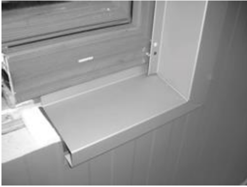
The window must be fitted with a bottom cill profile. The outside is sealed with a Type 8 vapour permeable sealing tape. This is covered by the sheet metal cladding.
